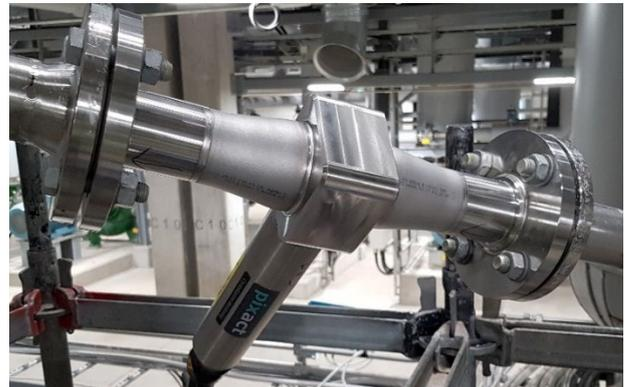
Figure 1. Installation of the PCM system on the crystallizer bypass line
